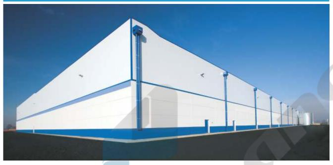
It is a double-steel sheet wall panel, insulated with polyisocianurate rigid foam. The tongue-and-grove joint is done using hidden through-fastened screw and saddle clip. External face available in Plissé, Box and Piano profiles. Internal face available in Box profile,
